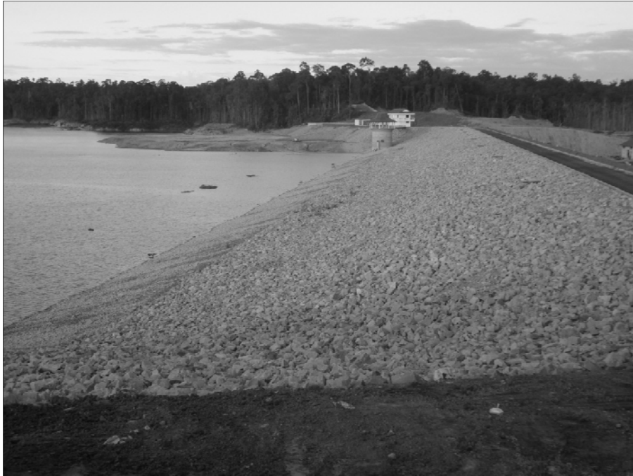
Figure 7. Photograph of Completed Embankment.
